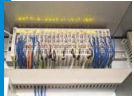
I/O – bus terminals (Fieldbus EtherCAT)
